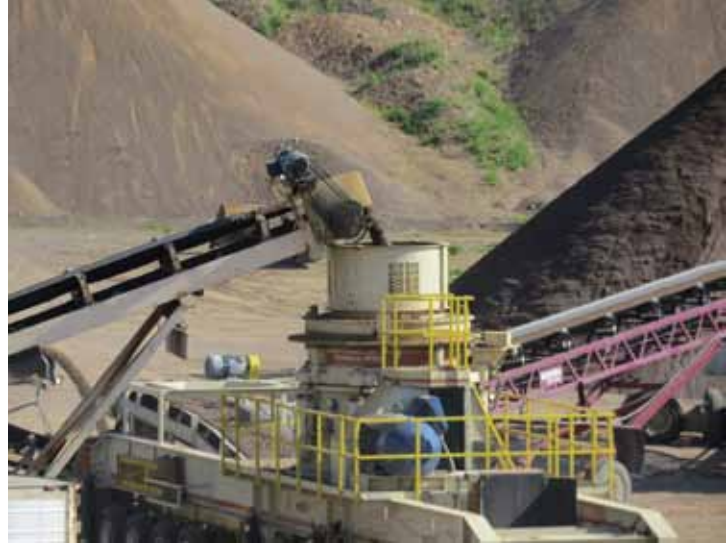
Crushing material using a Haas Cone Crusher.
