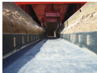
Belt Feeder with Canoe Liners on either side shown after 6 months of wear
