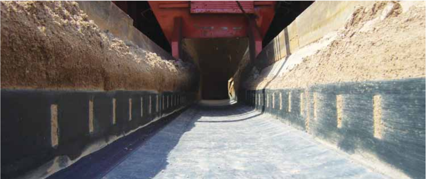
Belt Feeder with Canoe Liners on either side shown after 6 months of wear
